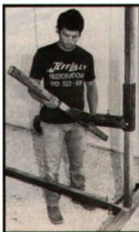
19 Attach the main center connector #10 to the outside connectors number #5.
